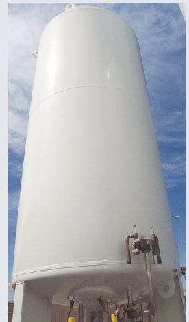
Cryogenic Bulk Tank
